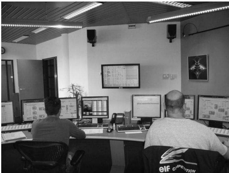
FIGURE 10. New control room, including overview display panel.
