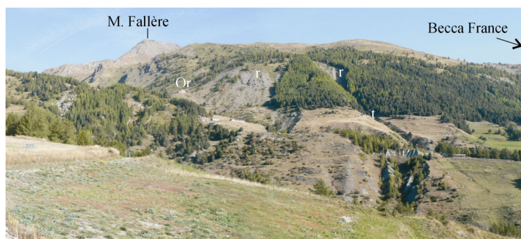
Fig. 11 - Extended area with very fractured rocks ( r ), connected to the P. Leysser DSGSD developed in the southern slope of the Becca France above the Or pasture. They may be confused with areas covered by debris sediments. A longitudinal trench, on the right, is deepened and enlarged by an ephemeral watercourse ( t ).
