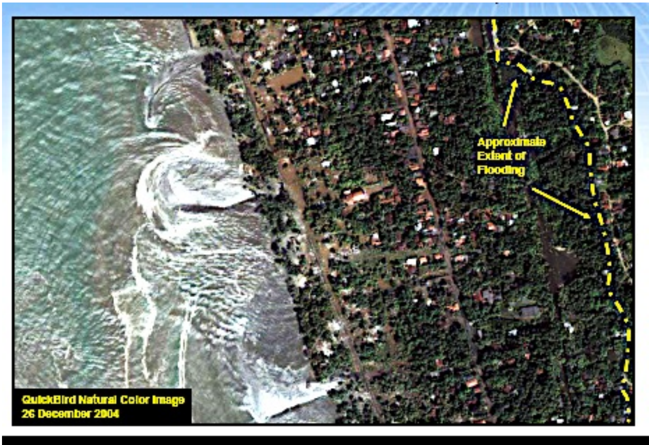
Figure 1. The Tsunami waterline: satellite view
