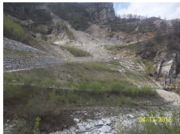
Figura 3.b: “Cava del Tiglio” Loc. Pra del Torno, in Rorà Village (TO), in this area it was used a “artificial loam” compared to natural soil and compost (at the bottom). (April 2012)
