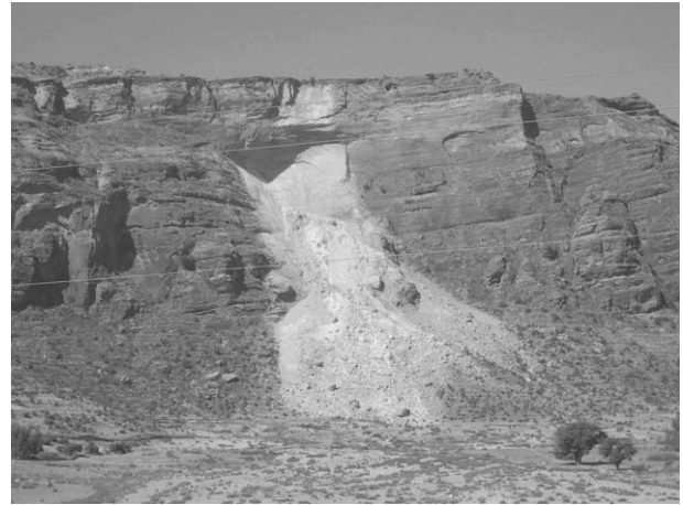
Fig. 8. A rock slide/avalanche involving the Adigrat Sandstone.
