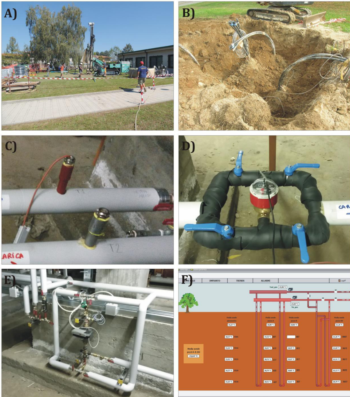
Fig. 8 – Pictures of the living lab. Drilling activity in front of the Topography department (A-B); temperature sensors placed throughout the circuit (C); ultrasonic flow meter (D); hydraulic circuit of the plant (E); underground section of the remote control system (F).
