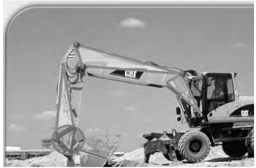
Fig. 2 - The excavator with flexible triangles and one flexible quadrilateral.
