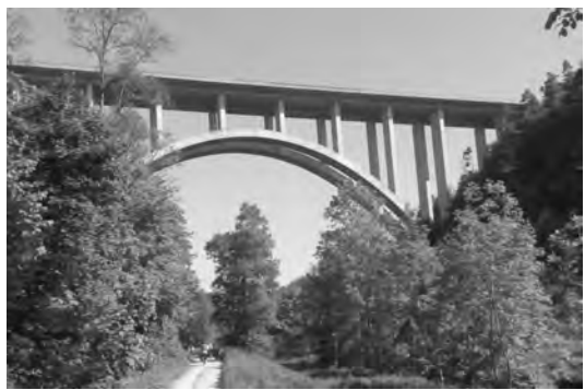
Fig. 14 - Bridge with a parabolic arc
