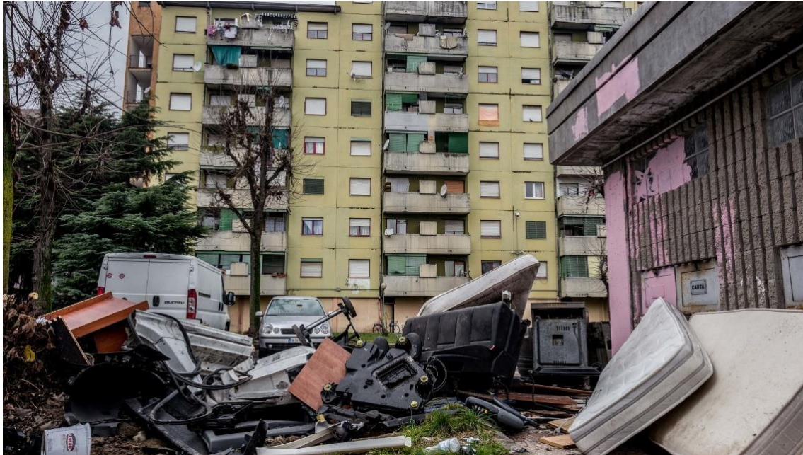
Figure 39. Abandoned objects in front of the yellow houses on Froth Street
