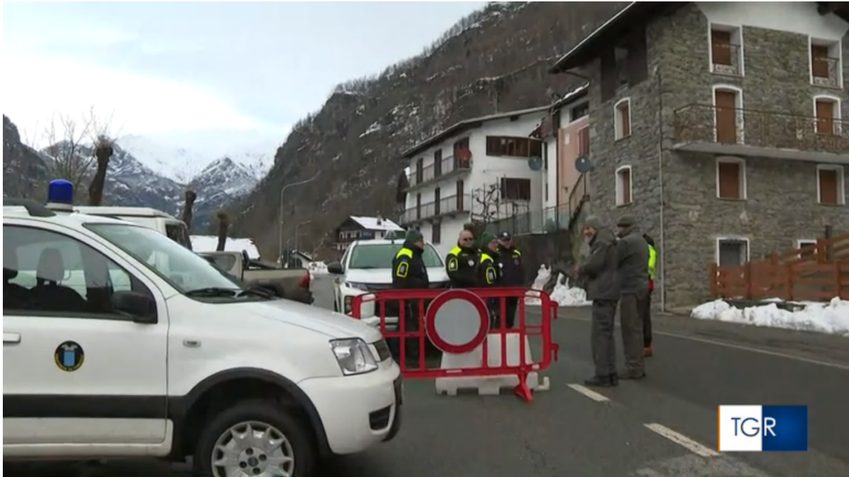
Figure 4-28: Provincial Road 299 blocked due to landslide (Source: RAI TGR)
