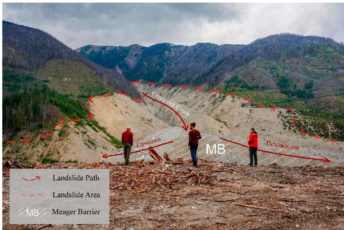
Figure 2. View to the northwest near the confluence of Capricorn and Meager creeks; Meager Creek barrier (MB) in the foreground. Part of the landslide travelled up Meager Creek (left side of image), but most of it travelled down Meager Creek to Lillooet River.
