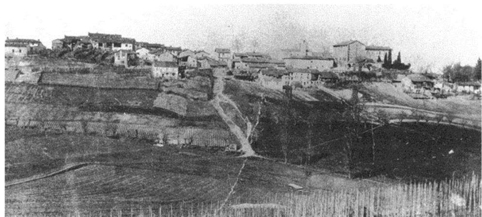
Figure 4. Coniolo hamlet in a photograph taken at the end of the 19th century. The village was abandoned, then completely demolished in 1907. Today, only few ruins of it are visible, called “Coniolo Rotto” (Broken Coniolo), hidden in a thick forest [46].
