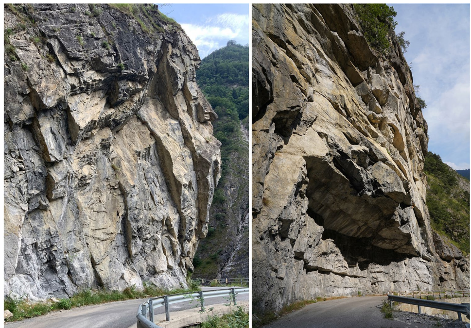
Fig. 5 Photographs of the rocky cliffs along the Elva valley road
