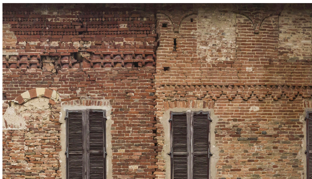
Figure 12. Section of the central part of the west front of the castle: on the left side, the earlier masonry and decorations (Period I), while on the right side, the connected masonry and Ghibelline decorations related to Period III.
