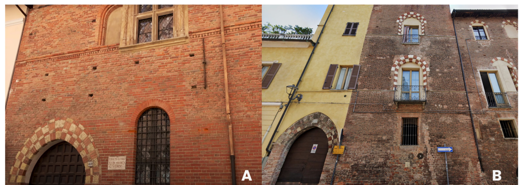
Figure 16. Comparisons on bichrome pointed arches related to doors and windows (ogival): (A) Verasis-Asinari Palace; (B) Roero Monteu Tower. From Google Street View.
