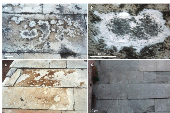
Figure 3. (a,b) BPs hypothetically related to previous lichen colonisation, and biofilm regrowth in their central areas (1990s); (c) BPs hypothetically related to lichen cover detachment (whitish surfaces) surrounded by brownish patinas (1990s); (d) BPs (whitish circular areas) hypothetically related to the past occurrence of lichen thalli, where the microbial recolonisation does not occur (2017). The block height is approximately 50 cm.
