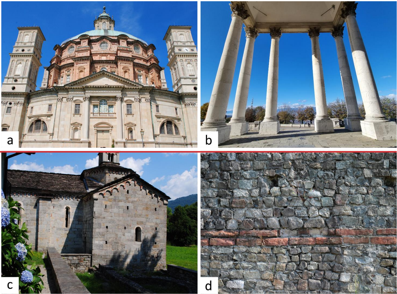
Fig. 43 Main examples of employment of Piemonte dimension stones in historic buildings: a) Sanctuary of Vicoforte built in Pietra di Vico; b) colonnade of the pronaos of the Basilica of Superga with several elements in Calcare di Gassino; c) Romanesque church of San Giovanni in Montorfano village built with the Granito di Montorfano; d) Eporedia (ancient Ivrea, Torino province ) amphitheatre wall mainly built with Diorite and Gabbro variety of the Granito Nero di Anzola
