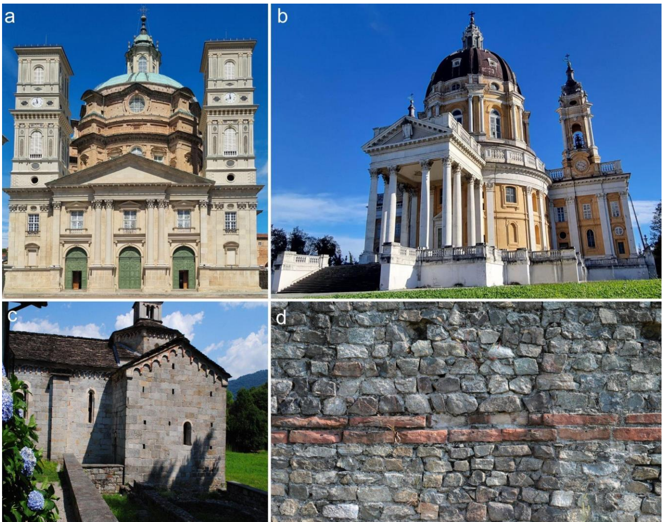
301 302 Fig. 4 Main examples of employment of Piemonte dimension stones in historic buildings: a) Sanctuary of Vicoforte built 303 in Pietra di Vico; b) Basilica of Superga with several elements in Calcare di Gassino; c) Romanesque church of San 304 Giovanni in Montorfano village built with the Granito di Montorfano; d) Eporedia (ancient Ivrea, Torino province) 305 amphitheatre wall mainly built with Diorite and Gabbro variety of the Granito Nero di Anzola
