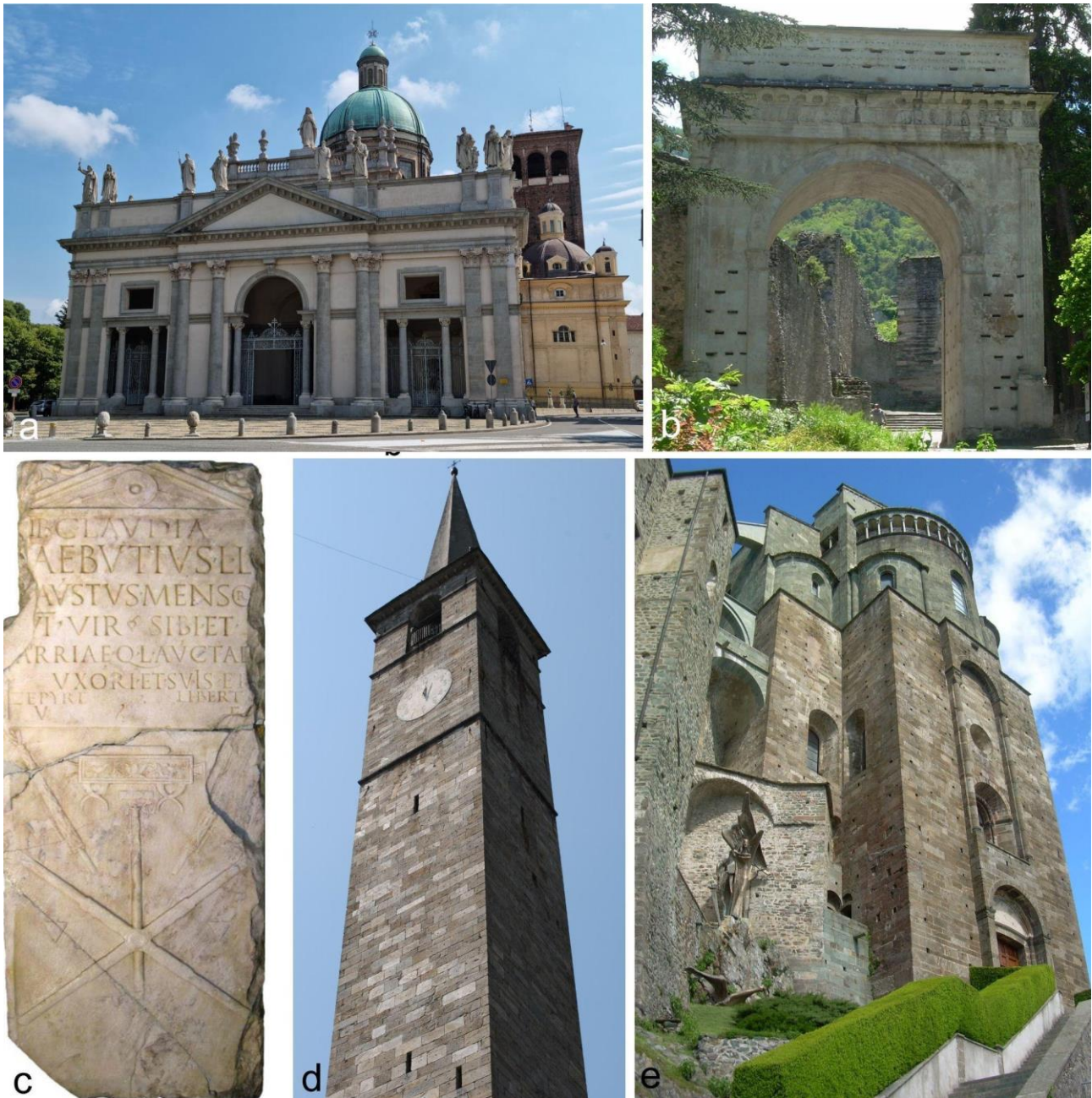
Fig. 7 a) Cathedral of Vercelli, in which Andesite del Chiavolino was used for columns; b) Arc of Augustus at Susa (Roman Age, 9 BC) built with the Foresto and Chianocco marbles; c) Funerary Stele of the Gromaticus carved using the Marmo di Pont Canavese and preserved at the Garda Museum of Ivrea (Torino); d) Santa Maria Assunta bell tower built in Serizzo at Montecrestese, Ossola Valley; e) Façade of the Sacra di San Michele made of serpentinite and metabasites
