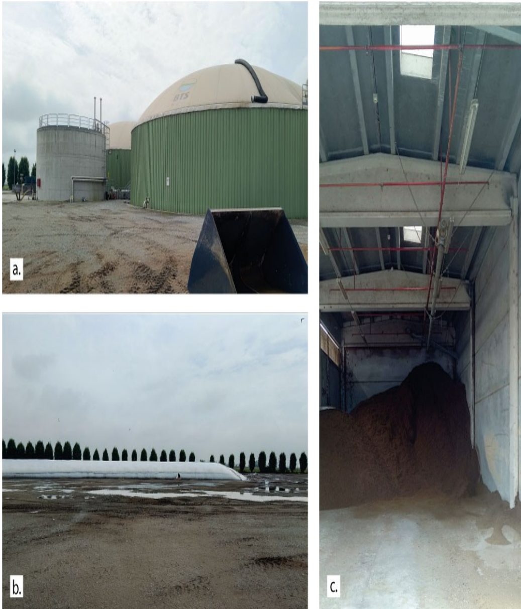
Figure 20: a) Agricultural biogas plant (ABP-3) that provided biomass samples for the experimental work; b) Silobag used for maize silage storage; c) Solid fraction of digestate on the storage platform.
