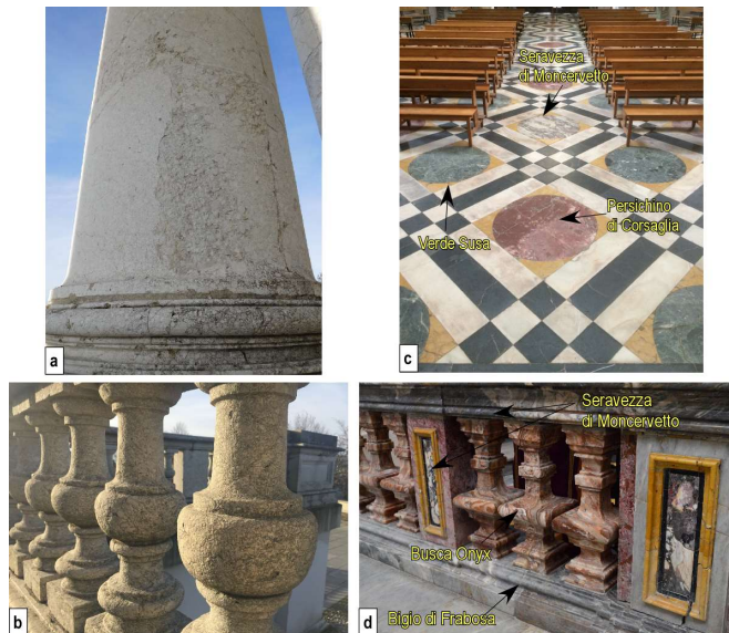
Figure 3.73: a. and b. Columns and pillars of balustrade of façade of the Basilica di Superga. c. and d. Interior pavement and balustrade of a chapel in which ornamental rocks used are highlighted.
