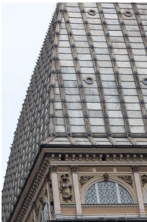
Figure 3.35: Detail of the slabs covering the dome of the Mole Antonelliana made up of Luserna Stone .
