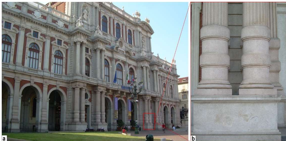
Figure 3.9: a. 19th century façade of Palazzo Carignano in Piazza Carlo Alberto in Torino b. Detail of columns made up of Baveno Granite .
