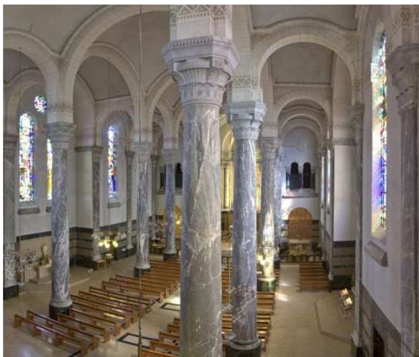
Figure 3.51: Monolithic columns and other decorations in Annecy Cathedral (France) made up of Bigio di Moncervetto marble.
