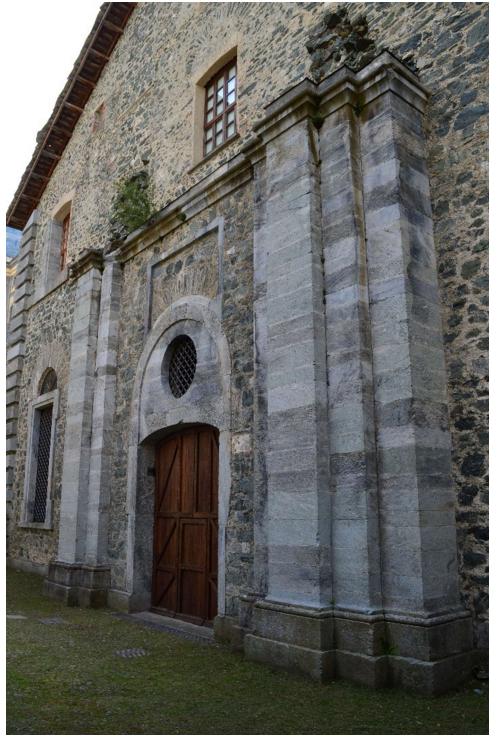
Figure 3.76: Detail of Porta Reale (San Carlo Fortress) in which calcschist is used for the pilasters and prasinite, metabasite and Malanaggio Stone for the wall.
