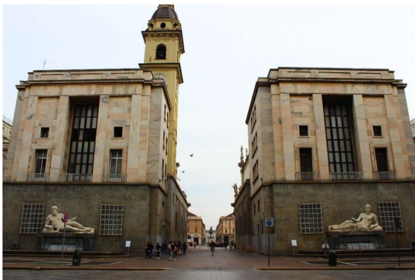
Figure 3.18: External coating of the apses of S. Cristina and S. Carlo churches in Piazza C.L.N. (Torino) made up of Ornavasso Marble .
