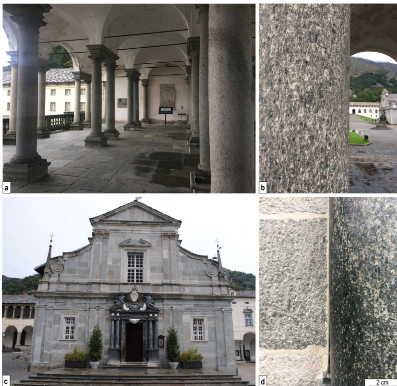
Figure 3.81: Oropa Sanctuary: a. Columns made up of Verde Oropa of the first courtyard and its detailed picture ( b. ); c. Old Basilica with façade made up of Verde Oropa and columns of the entrance made up of serpentized peridotite ( d. ).
