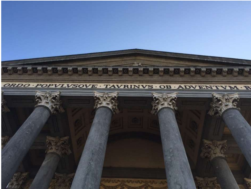
Figure 3.38: Columns of the façade of Gran Madre di Dio Church made up of Malanaggio Stone .
