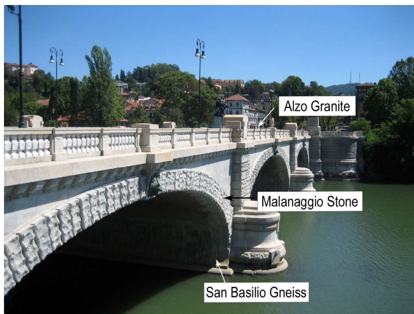
Figure 3.7: Umberto I bridge in Torino.
