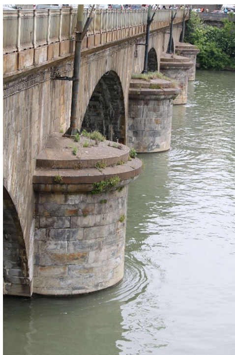
Figure 3.37: Detail of batteries coatings and the armlets of the arches of the Vittorio Emanuele I bridge made up of Cumiana Stone .
