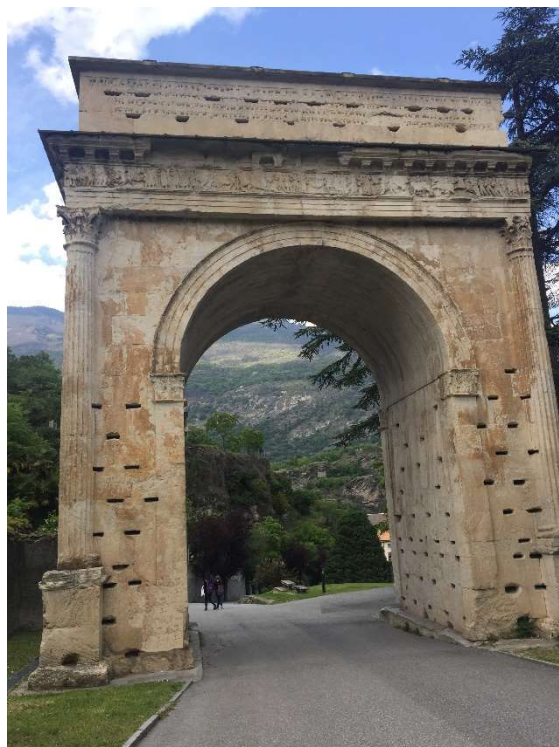
Figure 3.32: Arch of Augustus in Susa made up of Foresto and Chianocco Marbles .
