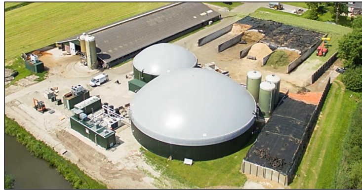
Figure 5: Example of an anaerobic digestion plant near a livestock farm.
