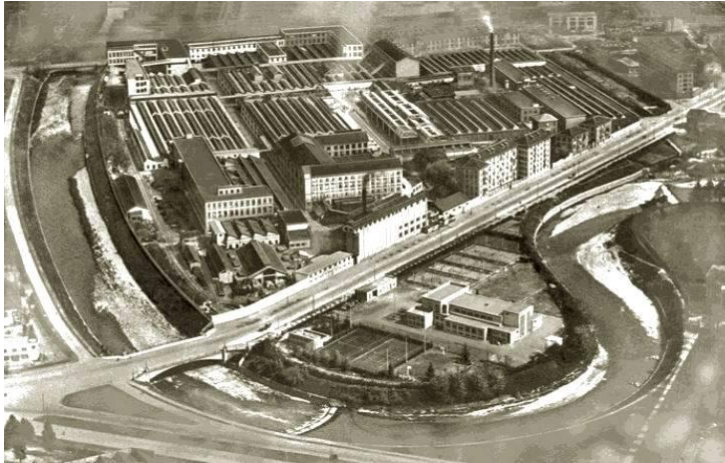
Figure 4.3a. Parco Dora as it was in 1950. Source: Comune di Torino.
