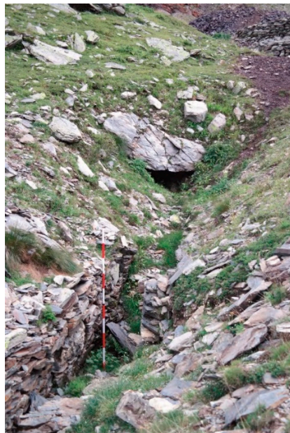
Figure 8. Piateda (SONDRIO), mining complex of Venina. View of the underground entrance to the mine with the access corridor outside (image by the Author).
