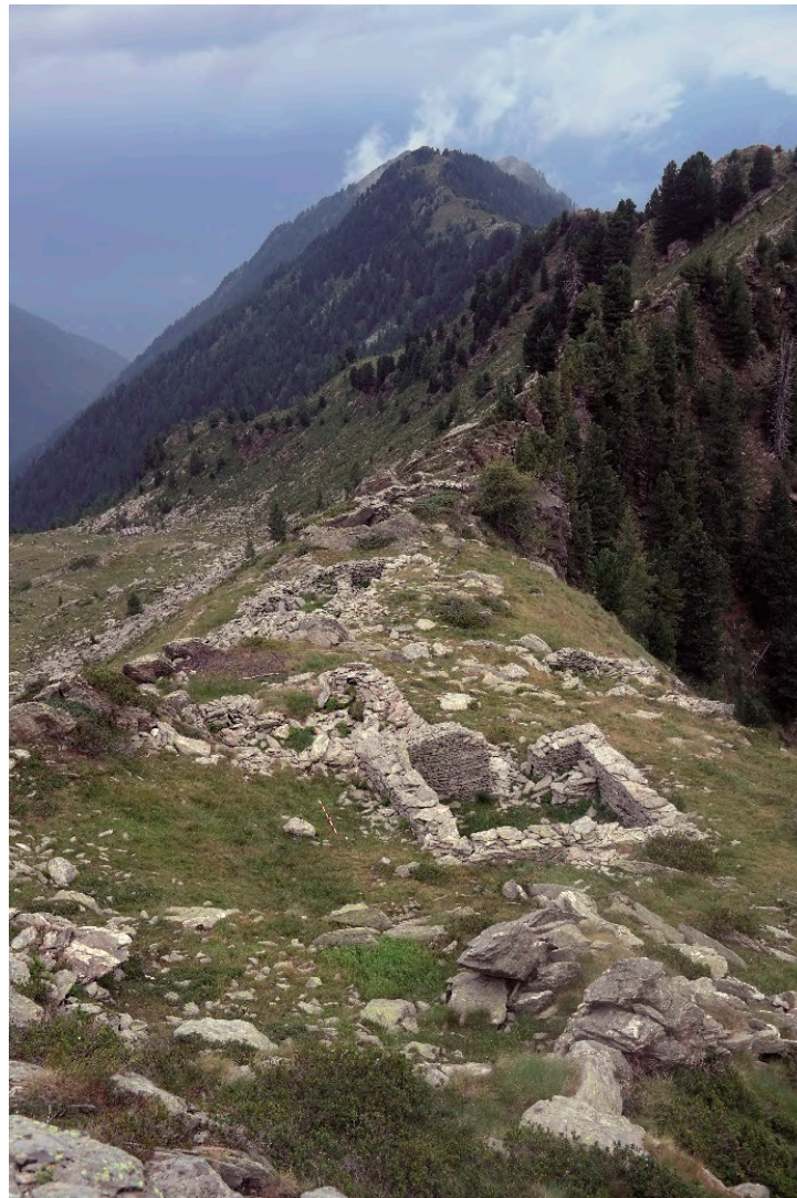
Figure 17. Fusine (SONDRIO), general view from the south of the miners' cabins on the watershed dividing Val Madre (on the left) from Val Cervia (on the right).
