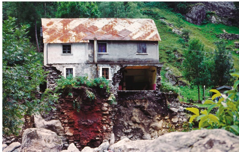
Figure 11. Vedello (SONDRIO), Privativa Tavelli damaged by the flood of 1987. Beneath the structure are the probable ruins of the smelting furnace which emerged during flooding when the Caronno river burst its banks (photograph by Marino Amonini).
