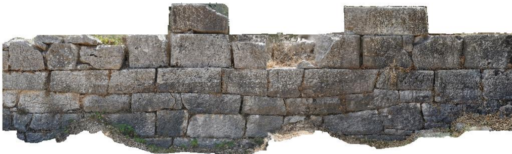
Figure 4.19. Orthoimage mosaic, cella wall remains at the Temple of Athena and Zeus Sotiros.
