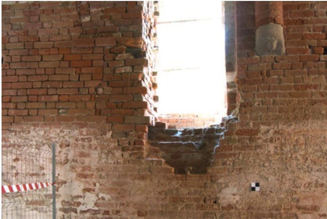
Figure 140. Detail of the removed pulpit on the south internal wall of the refectory (Photo F. Diara)
