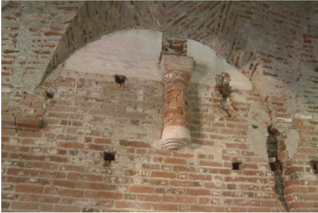
Figure 142. Detail of the semi-column related to the old ceiling on the north wall of the refectory (Photo F. Diara)
