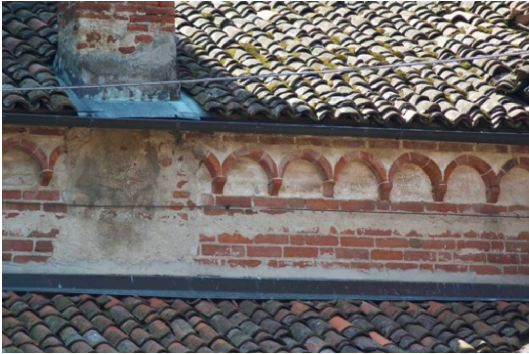
Figure 19. Protruding suspended arches on the external south front of the cloister, above the ceiling of gallery (photo F. Diara)
