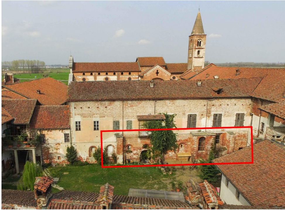
Figure 18. APR image of the external south front of the refectory. In red rectangle the refectory area (image from M. Roggero survey)
