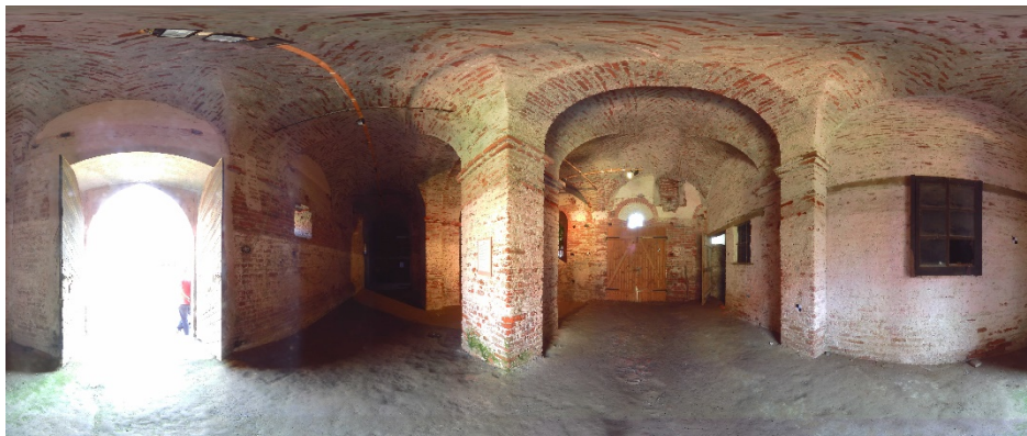
Figure 71. Panoramic image from laser scanner (2018 survey): inside the refectory
