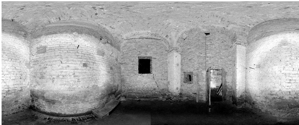
Figure 74. Panoramic image from laser scanner (2018 survey): inside the dark chamber
