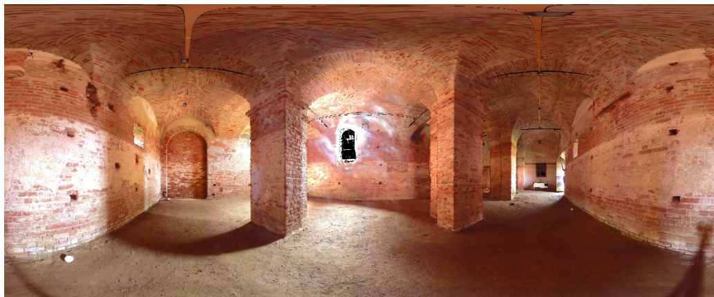
Figure 23. Panoramic image from LiDAR acquisition of the inside of the refectory (2): on left the north wall and partially the east wall with the covered opening; on right still the north wall and partially the west wall; in the middle part of the south wall (image from M. Roggero survey)
