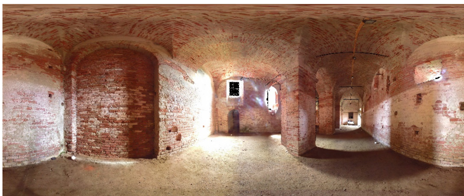
Figure 72. Panoramic image from laser scanner (2017 survey): inside the refectory
