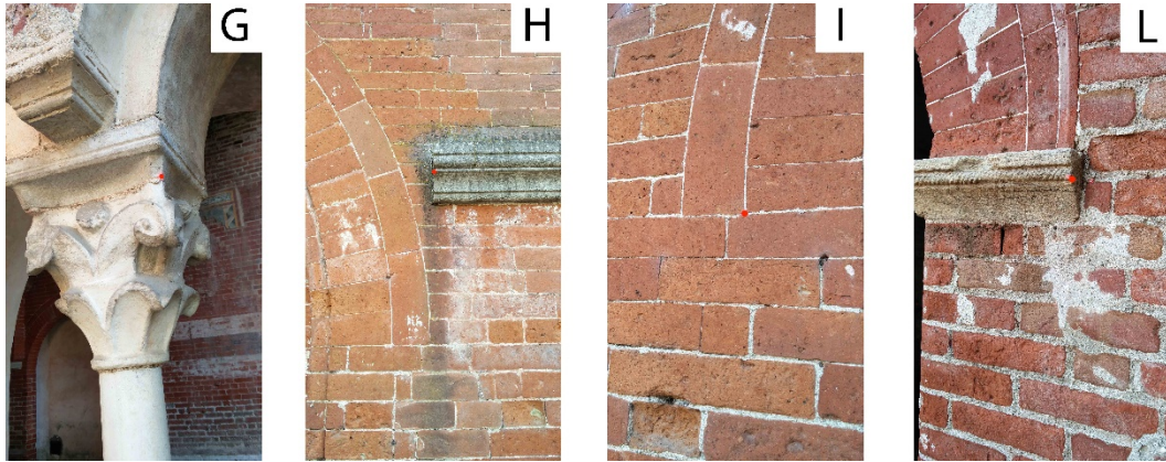
Figure 57. Natural points (red circle) registered on the cloister (3): G) point 7; H) point 8; I) point 9; L) point 10
