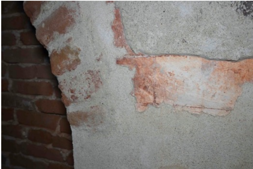
Figure 26. East wall of the refectory: detail of the earlier plaster that shows an imitation of bricks (photo F. Diara after a preliminary fresco restoration in 2019)
