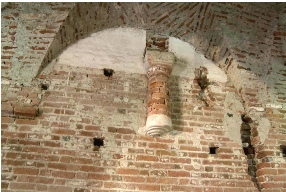
Figure 24. Detail of north wall of the refectory with a suspended semi column referred to the previous ceiling and the actual vaulted system (photo F. Diara)
