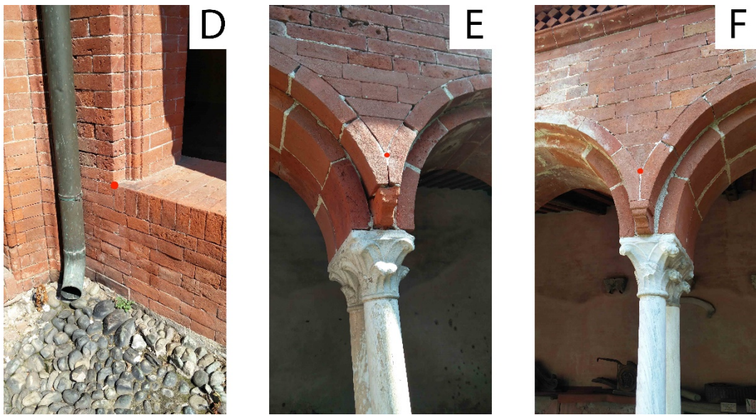
Figure 56. Natural points (red circle) registered on the cloister (2): D) point 4; E) point 5; F) point 6
