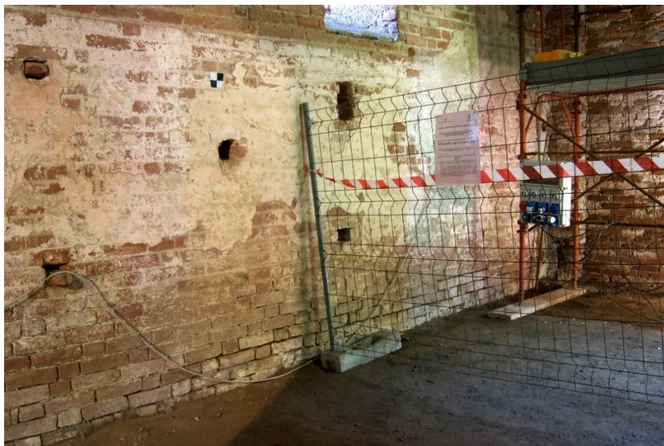
Figure 66. Image of north-east corner of the inner part of the refectory. On the right (east wall) can be noticed the restoration scaffolding (photo F. Diara)
