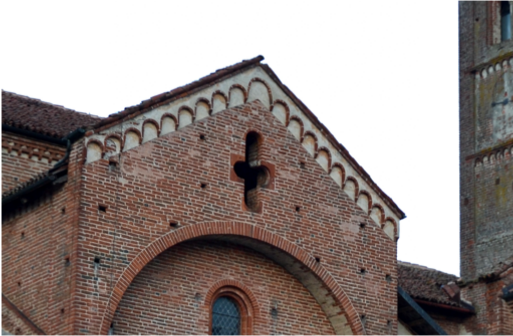
Figure 136. Suspended arches on the transept of the church (Photo F. Diara)
