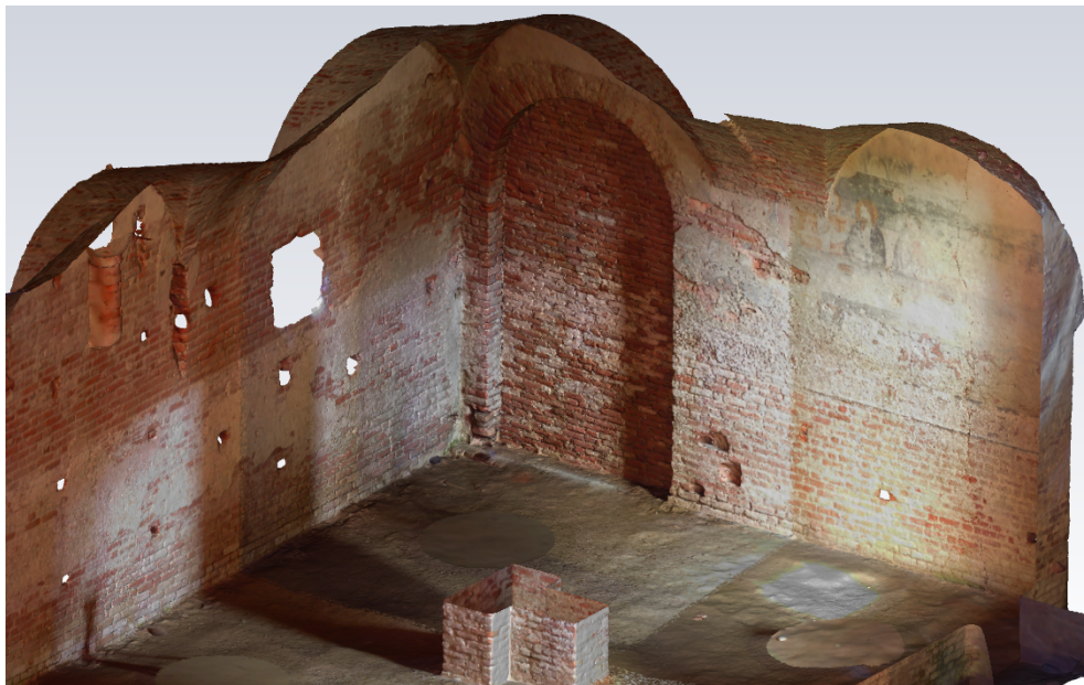
Figure 93. Radiometric values applied to the polygonal mesh (detail of south and east walls) - (elaboration F. Diara).
