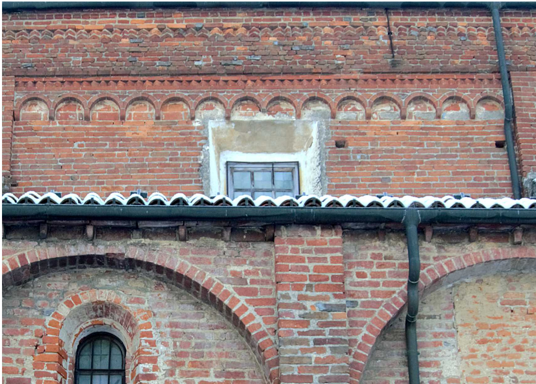
Figure 21. Casanova abbey: protruding medieval arches on the north side of the church (photo F. Diara)
