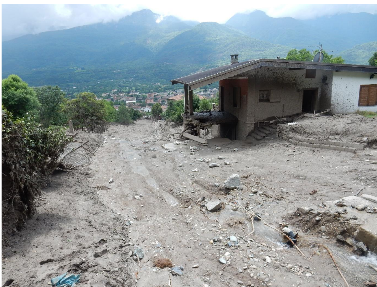
Figure 6.19 – Flow deposits and damages of the June 7 major debris flow at the Comba delle Foglie outlet (Bussoleno).
