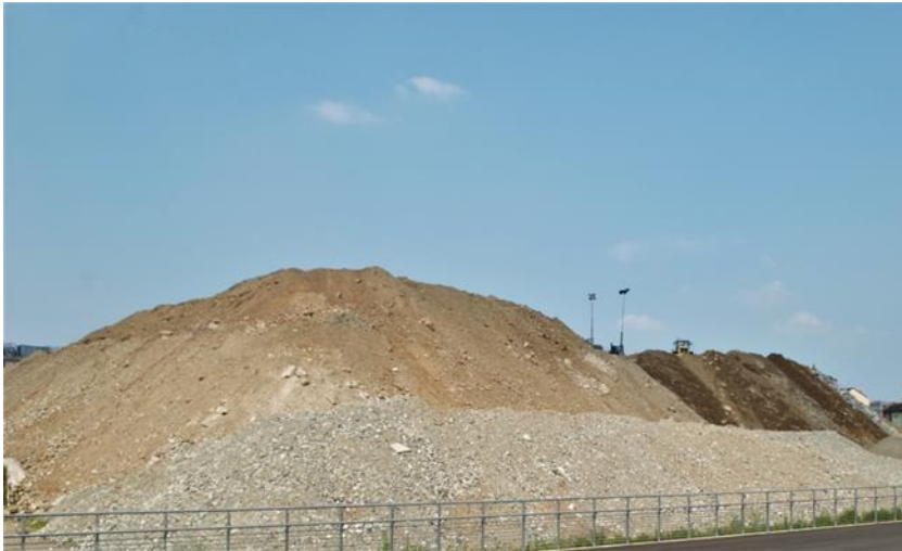
Fig. 4.4. Excavated material waiting to be redistributed. Foto by Ajmone F.
