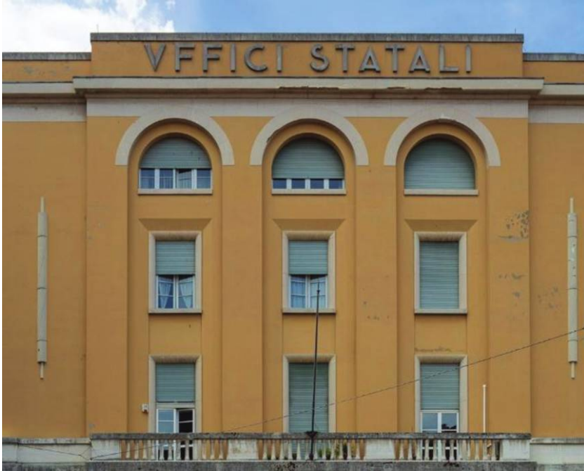
Figure 3. An example of typification through writings on the wall: the writing clarifies the type of the building (i.e., office building).
