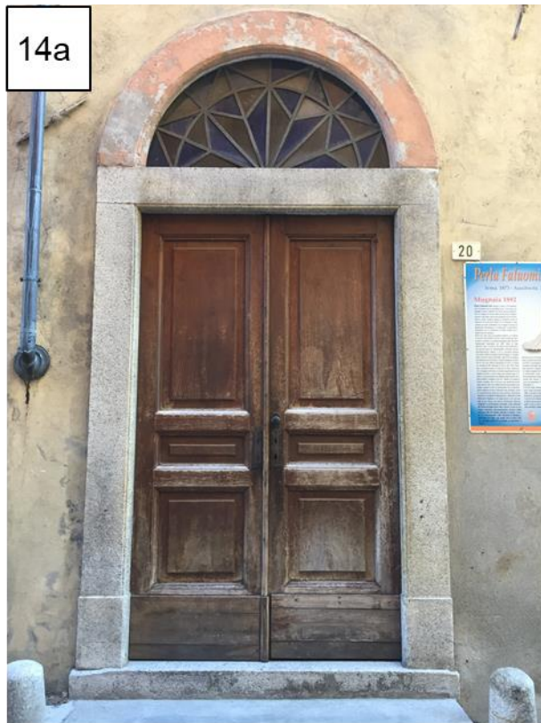
Fig. 14 stop 9: Entrance door of the Ivrea Synagogue (a): detail of the Montorfano Granite employed the entrance door frame; detail of the jadeitic orthogneiss for the access stairway
