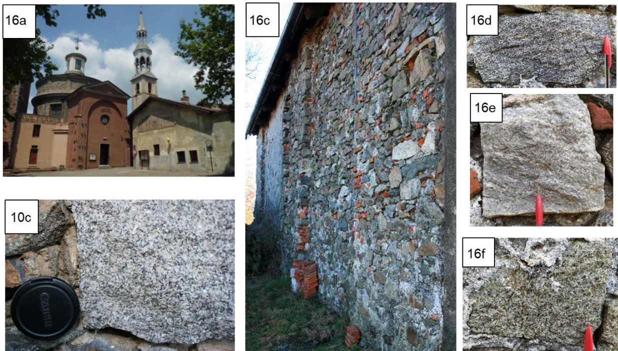
Fig. 164 Stop 12: Monte Stella Sanctuary (a); Detail of Diorite del Canavese used on the outside of the Sanctuary (b) ; Stop 13: medieval external masonry of Tre Re Chapel (c) ; Details of diorite (d), jadeitic orthogneiss (e) and serpentinite (f) of rock block employed in the masonry.
