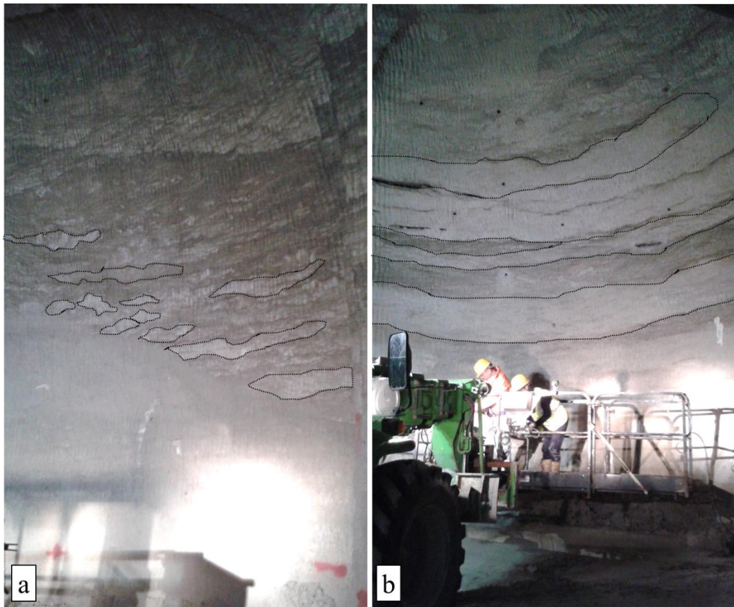
Figure 9.2 Excavation faces in underground tunnels in branching selenite gypsum with different macro-textural features. a. Small gypsum nodules in a predominant fine matrix. b. Big coarse gypsum branches with lower concentration of finer matrix.
