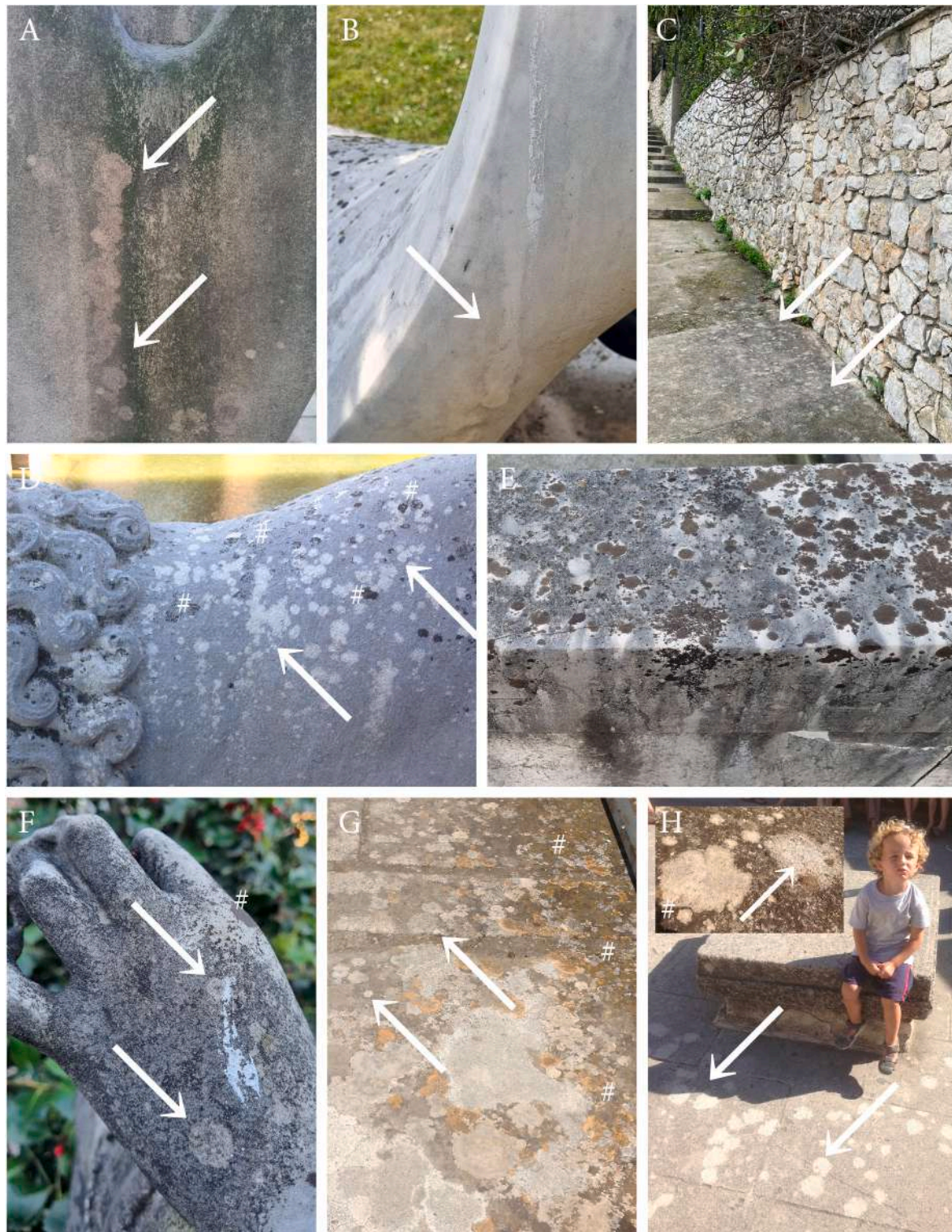
Fig. 1. The phenomenon of CUMBs observed on different stone surfaces. (A) Marble statue in the Monumental Cemetery of Milan (Italy); (B) marble statue in Parma (Italy); (C) cement pavement, beneath a fig tree, in Saint Jean Cap-Ferrat near Nice (France); (D) cement balustrade in the Kasteel de Haar near Utrecht (Netherlands); (E) marble balustrade and (F) marble statue in the Monumental Cemetery of Milan (Italy); (G–H) sandstone pavements of the walls of Aigues-Mortes (France; G) and of the Palace of the Popes in Avignon (France; H). Arrows indicate CUMBs; # indicate lichens in the nearby (in the inset in H).
