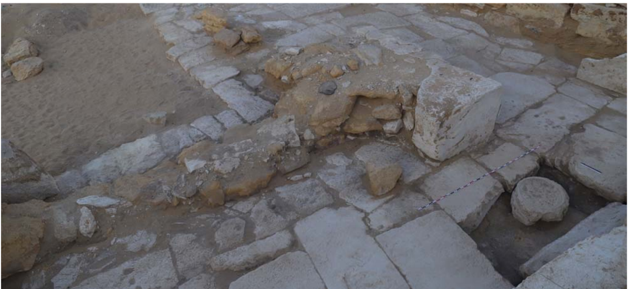
Fig. 9 - Southern corridor: view (from the North) of a portion of the inner wall, at the South-eastern corner. The photo shows the emplekton technique used for the wall building (photo: M. Nuzzolo)
