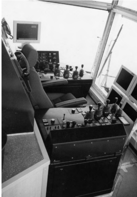
FIGURE 12. Heating radiator located exactly at the best standing position for a lock master.
