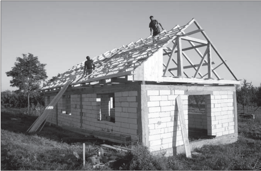
Image 4. Roma building a new house.
