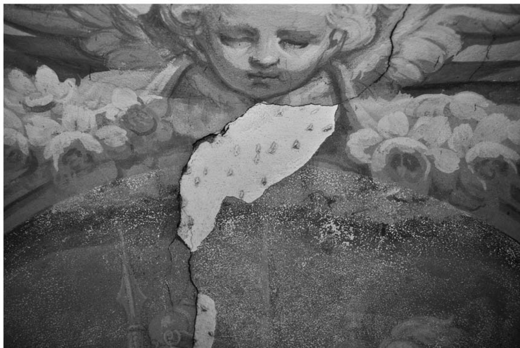
Figure 4. In the picture it is clearly observable the whitish surface of the mid '700 plaster, which was lately in mid '800 scaled with hammer to obtain a rough surface for a better adhesion of the new mortar and pictorial decoration. FOV 40 cm.
