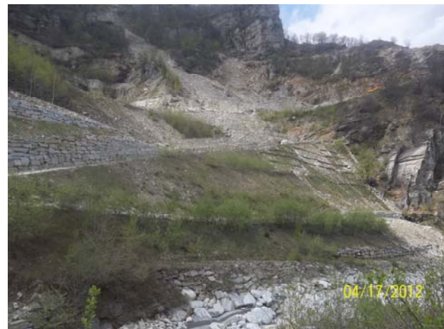
Figura 3.b: “Cava del Tiglio” Loc. Pra del Torno, in Rorà Village (TO), in this area it was used a “artificial loam” compared to natural soil and compost (at the bottom). (April 2012)
