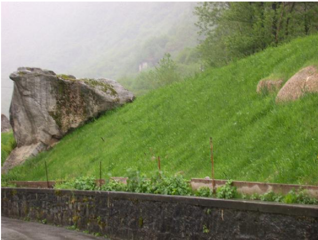
Figure 1: Loc. Lodrino (Canton Ticino), in this area it was used a “artificial loam” obtained from a bioremediation treatment, after some months from the seeding
