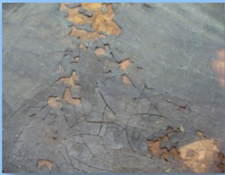
Cracking and lifting
