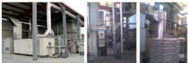
Figure 3. Some energy generators (left picture: gasifier) and loads (right pictures: process machineries) of the demo site.
