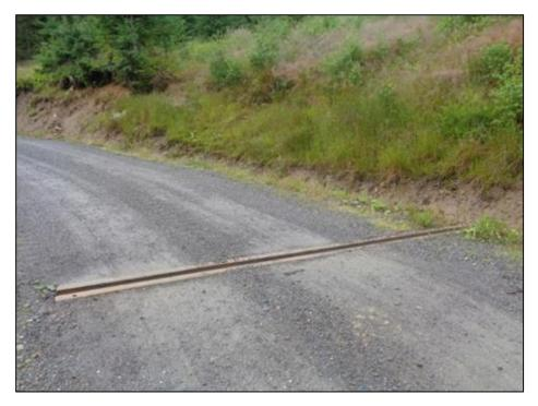
Figure 29. Device used to disperse the surface runoff in order to reduce erosion of the slopes.
