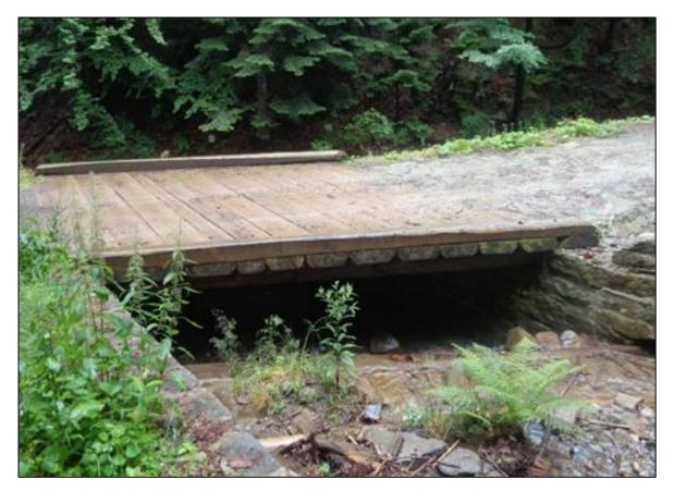
Figure 31. Wooden bridge more user friendly to aquatic organisms replacing concrete culvert.
