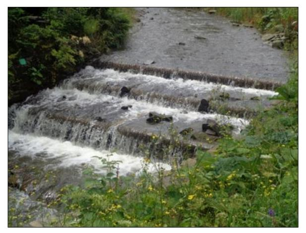
Figure 30. Wooden steps reducing the slope of the torrent but not blocking the movement of aquatic organisms.
