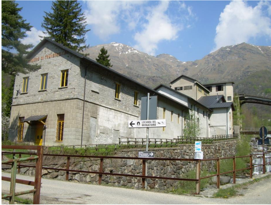
Figure 22. Dressing plant, now abandoned and partially used for the Museum of Minerals and Equipment of Traversella Mine
