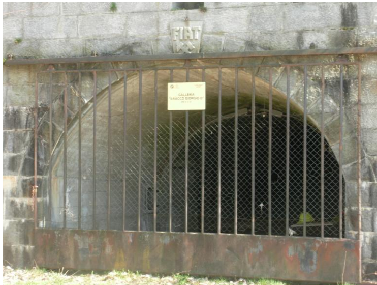
Figure 19. Entrance of an old tunnel (Galleria Bracco Giorgio D)
