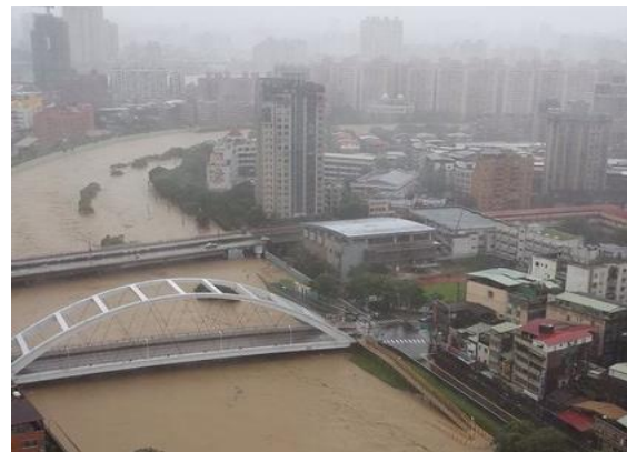
Fig. 2. The soared flood of Jingmei River caused by Typhoon Sudeil. Source: http://www.appledaily.com.tw/realtimeneews/article/new/20150808/665238/
