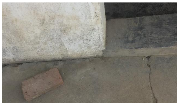
Fig. 7. Reconstruction house with concrete rather than clay.
