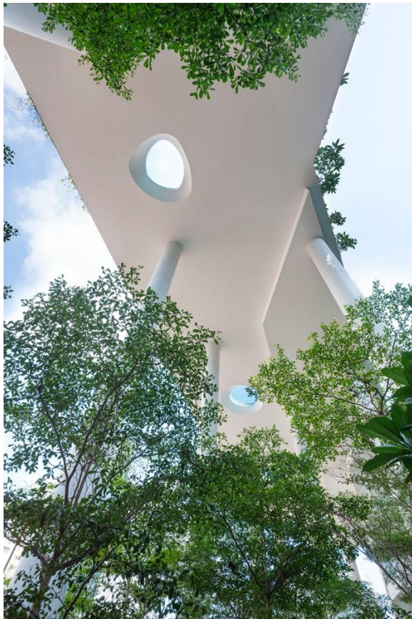
Fig 13. An urban forest of trees reaches out from the 1 st storey landscape terrace to the cantilevered pool overhead. An amorphous-shaped skylight frames a piece of the sky. Photo by John Gollings; John Gollings Photography
