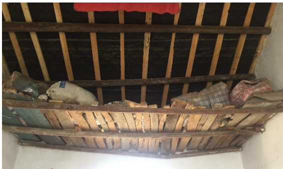
Fig. 5. Extra shelf for storage during the flood.
