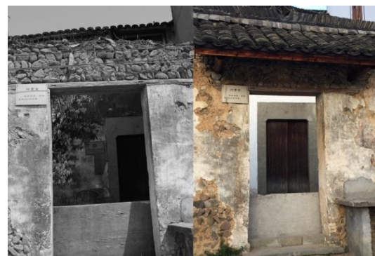
Pic. 13 Repair of building facade at the entrance of Xingsu
