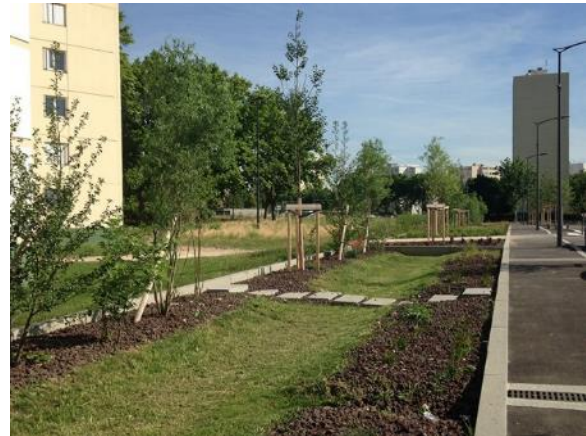
Fig 6 – The rainwater management of all local streets in the urban zone is exclusively alternative via rain gardens or ditches. This sector’s construction ended in 2015.
