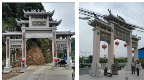
Fig. 5 Memorial archways of Datian and Jingnan, Fujian province, China.
