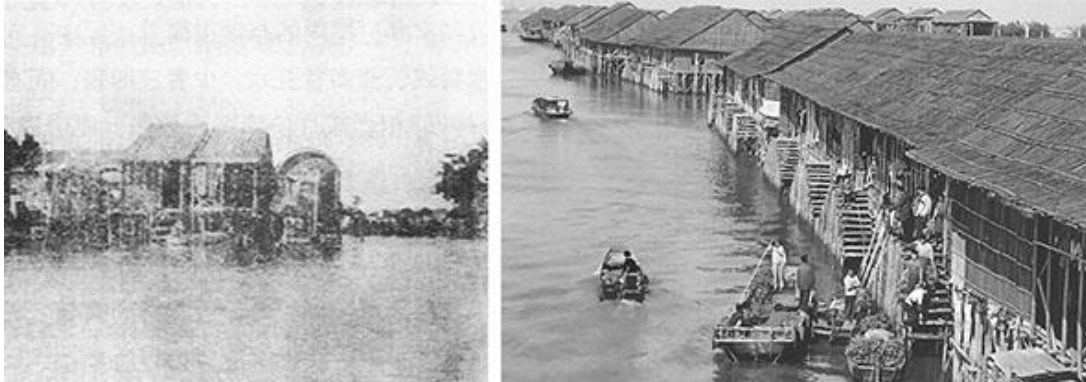
Fig. 9. Residential building standing on the wood pillar. Left one is the simple shed standing on the water in the Republic of China era and the right one are buildings in Wanqingsha Island which facing the waterway and have wooden stairs to access water front.
