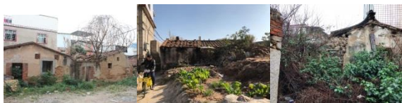
Fig 14 abandoned historical buildings
