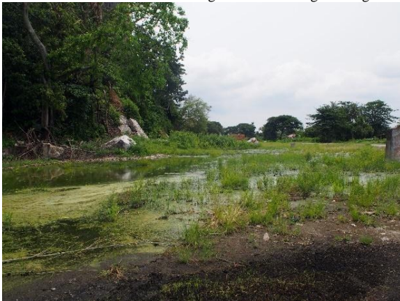
The water stagnant due to improper storm water management
