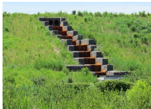
Figure 9 : Storm water is collected via a network of storm water swales, channels, and down chutes Source: http://freshkillspark.org
