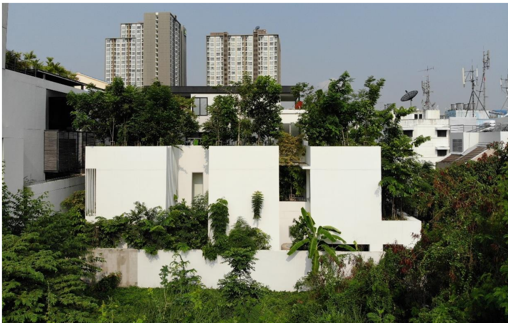
months after completion
