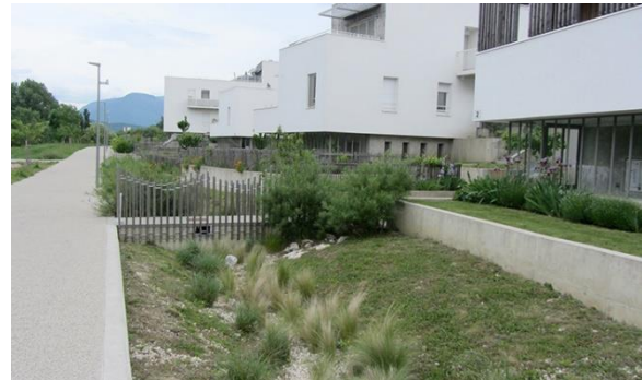
Fig.12. Wide planted gap separating private domain and the public path rainwater ditch.
