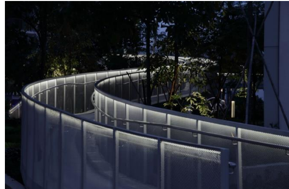
Fig 6. A mesh walkway weaves between trees in curvilinear form. Photo by Takeo Sugamata; SWITCH
