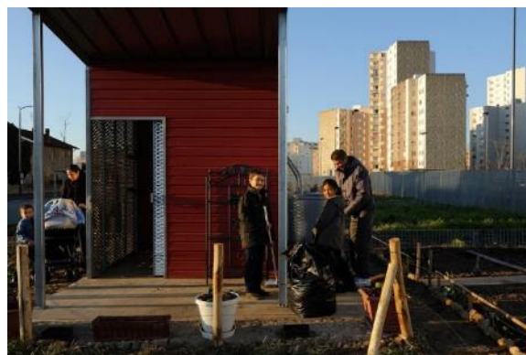
Fig 3 – The building of a garden shed in the Ecoin neighborhood communal gardens
