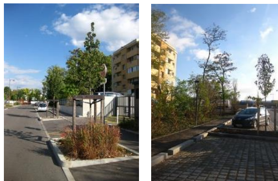
Fig 10 – Planted street with permeable surfaced parking. End of project construction: 2015
