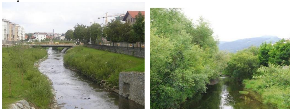
Canal Artia Irun-Spain-One of the works to be analyzed by SCIA SL in ECOMED Project G. Vasco P. Sangalli AEIP EFIB
