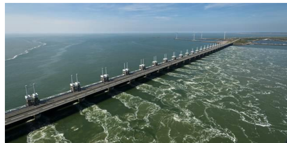
Fig. 1. Oosterscheldekering, an open barrier construction (sea on the left of the barrier) photographed during flood tides, The Netherlands. © maritimnieuws, RWS
