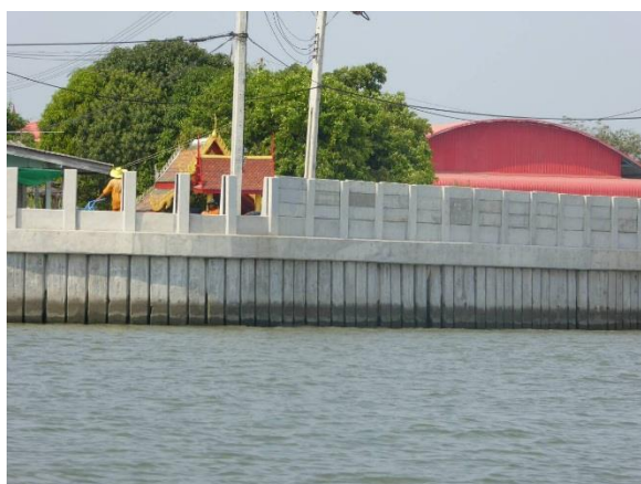
Fig 6 Floodwall along Chaopraya River
