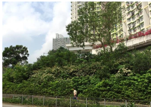
Fig.12b. After restoration in 2015: Lush vegetation with multiple strata of high ecological value
