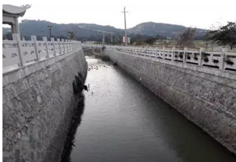
Fig. 7. Cement barriers of the river , Huian, Fujian province, China.
