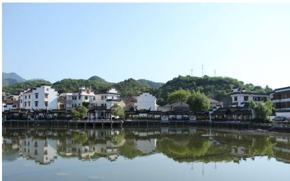
Pic. 12 The ancient village and skyline after the control of appearance
