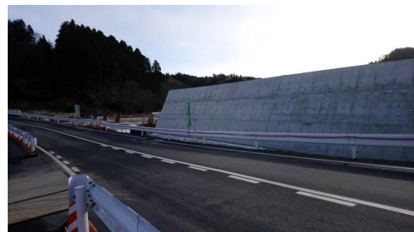
Fig. 5. Construction of Route398/seawall (Dec, 2017)
