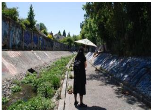
Fig. 6. A resident strolls along a creek maintenance road imagining possibilities.
