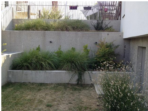
Fig.11. The carpark “green wall”
