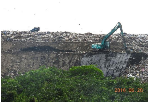
Figure 11: Slope stabilization process Source: Karadiyāna waste management facility
