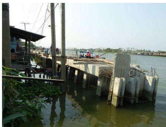
Fig 7 Construction of Floodwall along Chaopraya River
