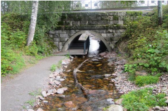
Fig. 4 The tunnel with a pier for pedestrians
