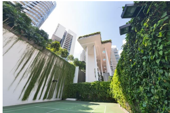
Fig 14. Nature takes over architecture, with creeper plants cascading down a high wall on one side and creeper plants forming a thick green wall around the tennis court. Photo by John Gollings; John Gollings Photography
