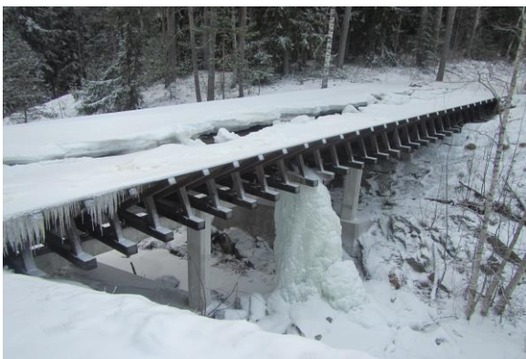
Fig.5 The aqueduct in winter
