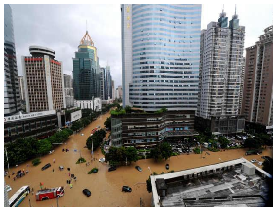
Fig. 3. The flooding of Fuzhou City caused by Typhoon Sudeil. Source: http://www.appledaily.com.tw/realtimeneews/article/new/20150809/665974/
