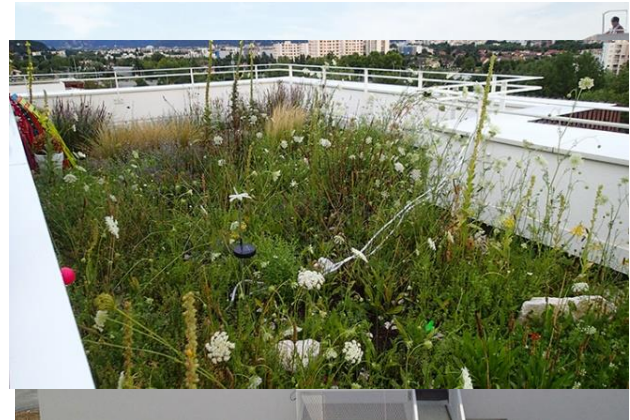
Fig.8. Extensive green roof just after planting
