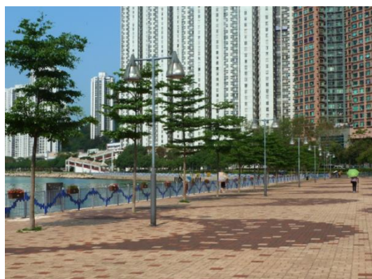
Fig.19. Enhancing the streetscape of our community through greening, design and selection of paving patterns and street furniture commensurate with the environment
