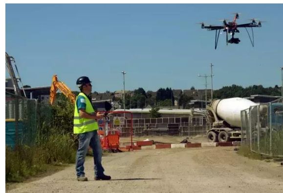
Fig. 3. Construction management supervision by UAV.
