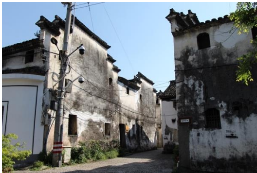
Pic. 9 Anhui Architecture with white wall and grey tiles, corbel-steps above the roof
