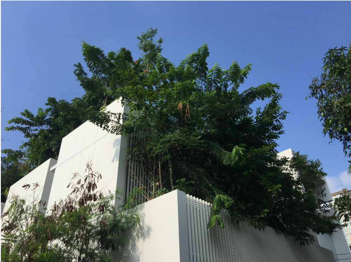
10 months after completion
