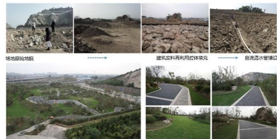
Fig.10. Xiang Wang road node sponge green space construction process and completion effect.
