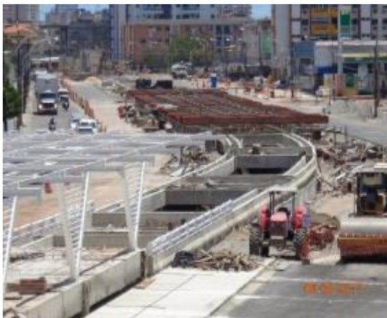
Fig. 1. Bus rapid transit corridor construction above Aguanambi Canal
