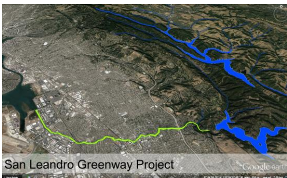
Fig. 3. The San Leandro Creek flows across East Oakland as the only remaining entirely day-lighted watershed in the city.
