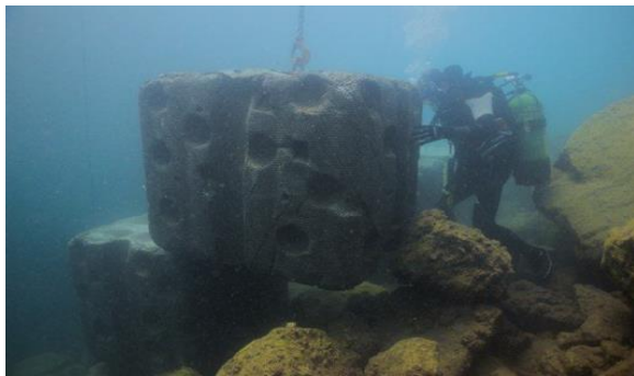
2013) ECONcrete®Antifers (EA) undergoing deployment by a technical dive team.(Blue is the new green – Ecological enhancement of concrete based)
