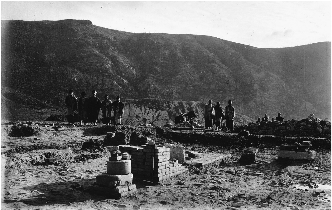
Fig. 8. Kal-e Chendar. Baked brick structure discovered by A. Stein ( Stein 1940. fig. 53)
