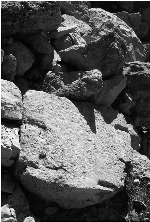
Fig. 14. Bilevah. Stone block of masonry with carved recesses for iron clamps (© Centro Scavi Torino and ICAR)
