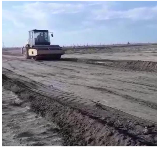
Figure 11. Compaction of the stabilized soil layer.
