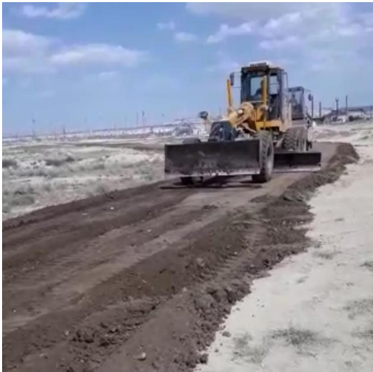
366 Figure 10. Levelling of the stabilized soil layer.
