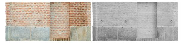
**Figure 12.** Comparison of details from the VIS (**left**) and NIR (**right**) dataset 2 textured models to evaluate identification of bio-deterioration on the façade's surface.
