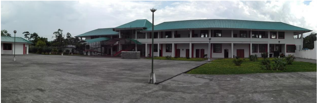
A school building in the Ahuano Millennium School we visited (Anu Häkkinen 2015)
