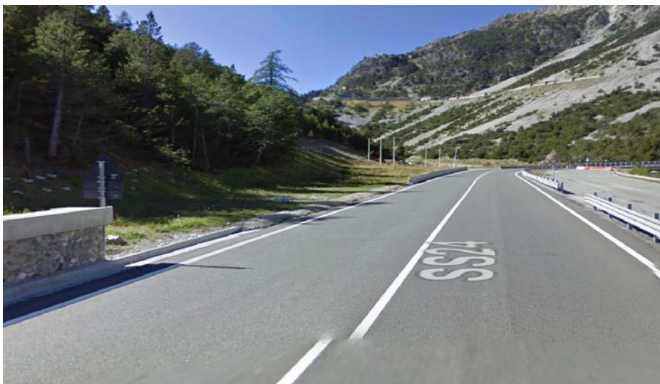
Figure 4 - View of the asset at stake – Road SS24.
