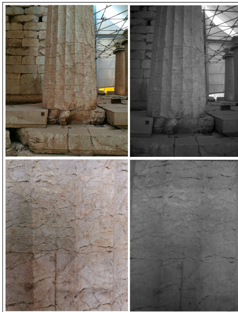
Figure 4. Color ( left ) and near-infrared reflectance ( right ) images of the same column captured at the Temple of Apollo Epikourios at Bassae, from further and closer range.
