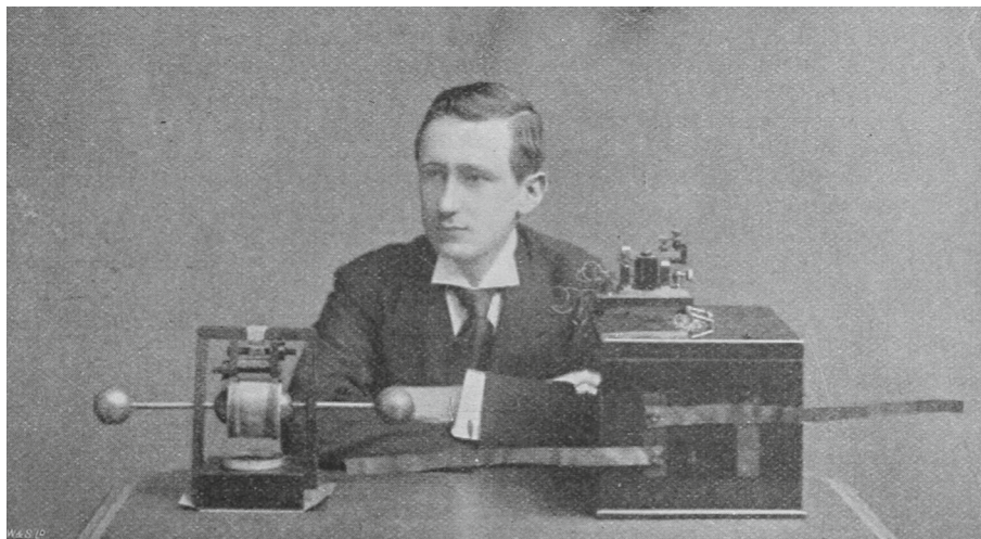
Fig. 2 Marconi with his instruments [21]. At left, one can see Marconi’s transmitter. Marconi’s receiver is inside the closed box
