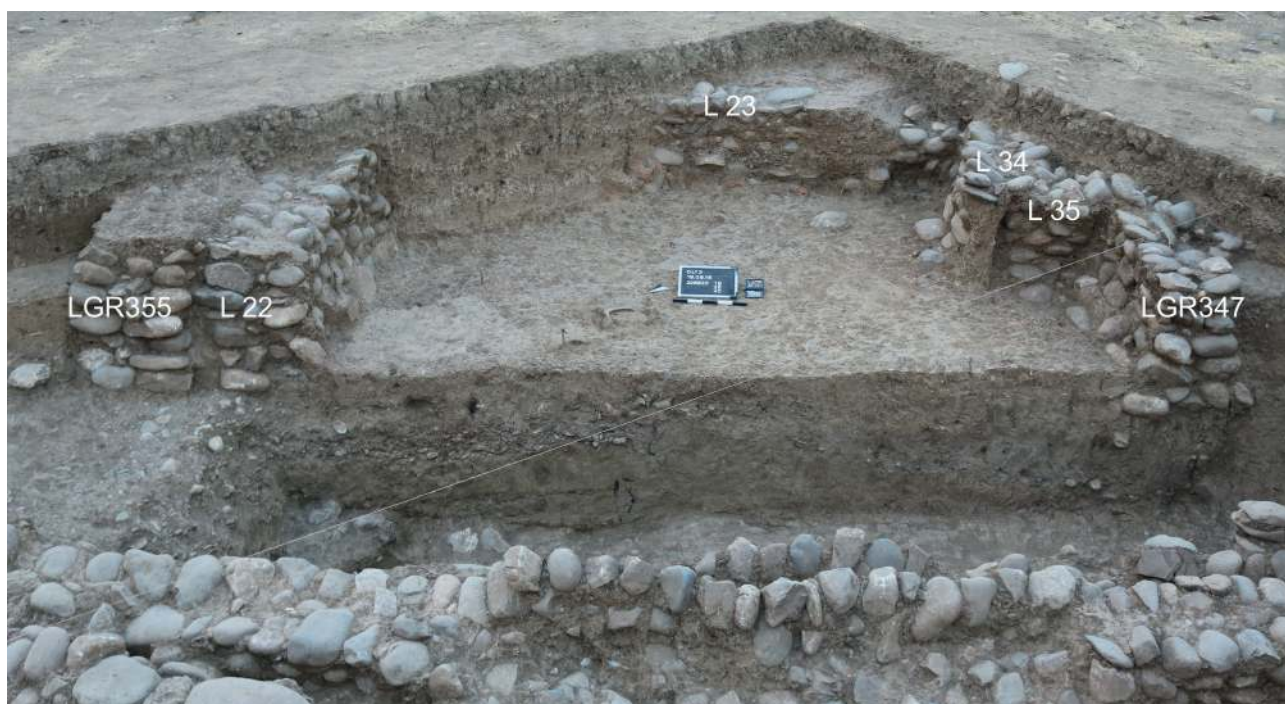
Fig. E14: Room 64 / Building R, view from the northwest. Photo by Jens Rohde, annotated by Andrea Squitieri.
