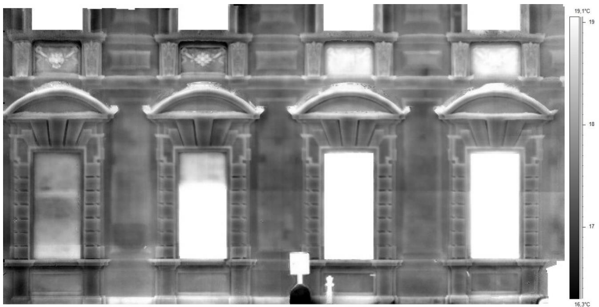
Figure 5.11. Thermal orthophoto-mosaic produced with FLIR 660SC imagery.
