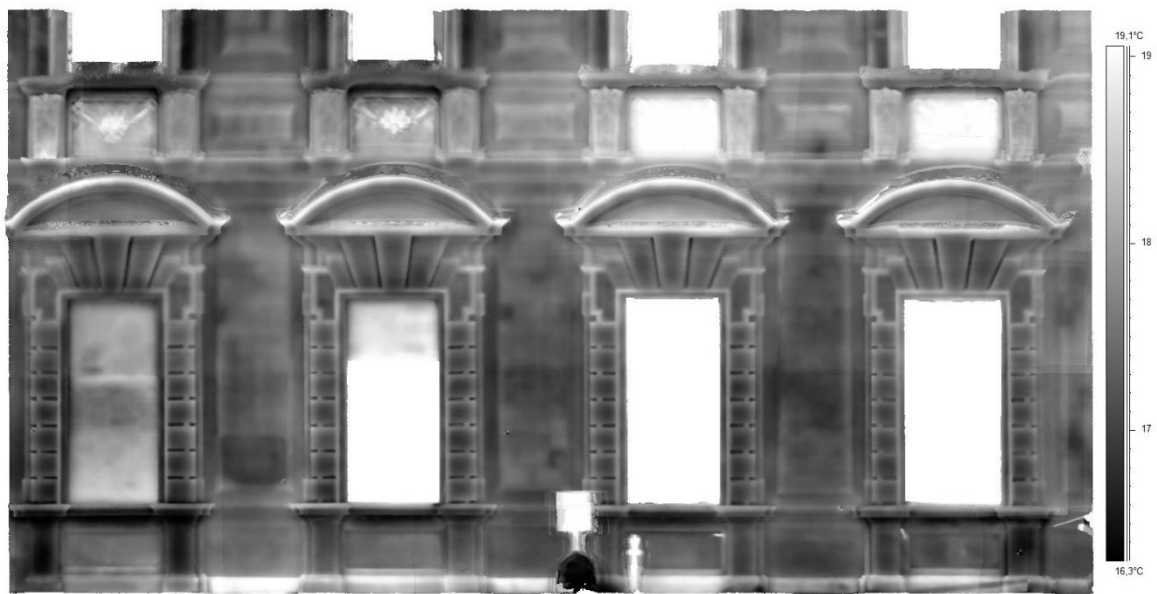
Figure 5.5. View of the façade's model with thermal texture.
