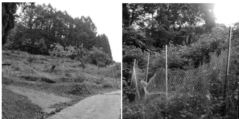
Figure 2. Collapsing macaque-proof electric fences (in Aomori prefecture, northernmost mainland of Japan). Although these fences can prevent against macaque intrusion into farmland, the steep terrain surrounding the farmland and inclement weather condition (e.g., typhoon, heavy snowfall) make it more difficult for the owners (i.e., farmers) to maintain the fences in good condition.
