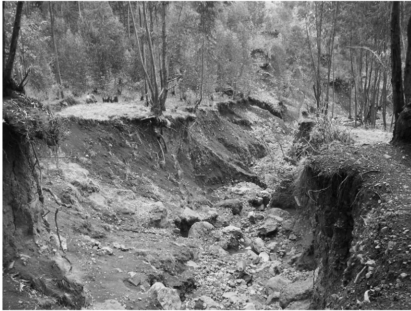
Fig. 9. Tossa talus belt with a landslide trench.
