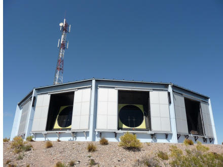
Figure 6: FD building at Los Leones during the day. Behind the building is a communication tower. This photo was taken during daytime when shutters were opened because of maintenance.
