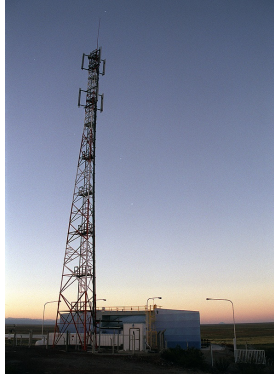
Figure 12: One of the five communications towers: the one shown is deployed at the Los Leones site; see Figure 11.
